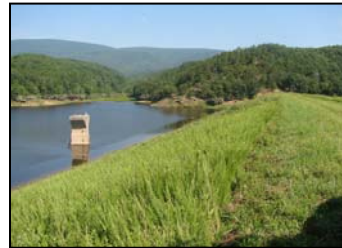
Dam #1 Summer of 2006
