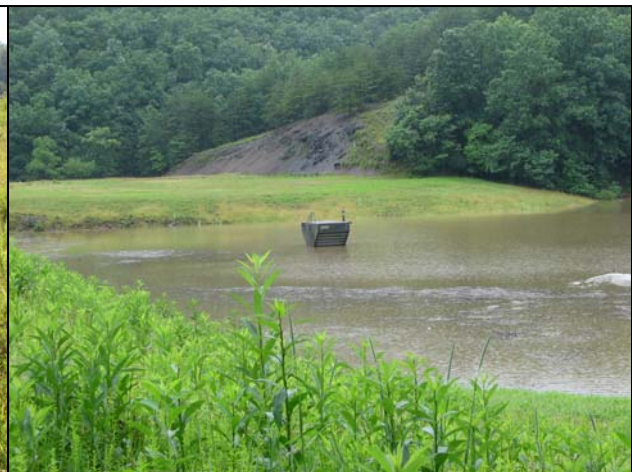
Dam #4 after a flood in Nov. 2006
