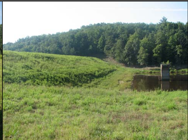
Dam #2 during the summer of 2006
