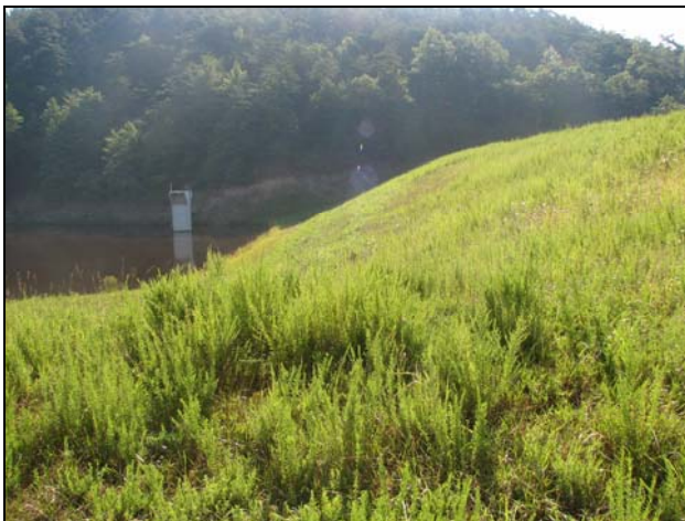
Dam #3 during the summer of 2006
