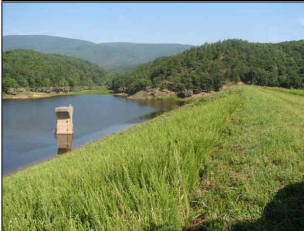
Dam #1 during the summer of 2006
